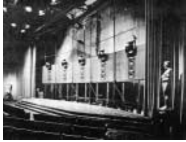
Figure 5: Theater Speaker Array at MGM[8]
